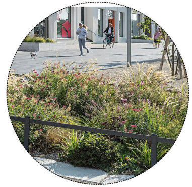
Abb. 11: Retentionsbeet
